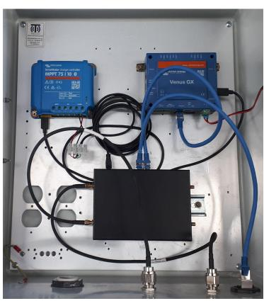
high speed data access in remote or low signal areas, powered via a solar panel. There is plenty of room to maneuver the X1 Pro to fit additional equipment. Optionally, a long range WiFi hotspot can be created by connecting the WiFi antennas on the right hand side to suitable external antennas; or a localised hotspot for administration of the box can be created by attaching the included WiFi antennas inside the box, as the box is made of plastic.
